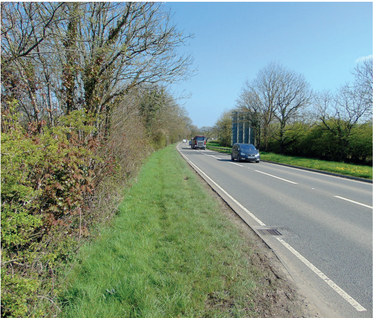
Figure 4: The existing A40 trunk road, looking east
