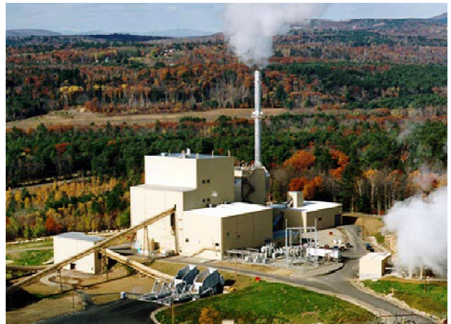
A 35 MW biomass power station in the US
