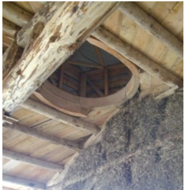
One of the roof lights under construction
